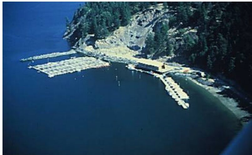
Figure 2: Pens located inside Shoal Bay at Lopez Island in 1980, with breakwater (upper left) partially preventing water circulation.
